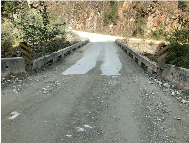
Left Bank Abutment when facing downstream
