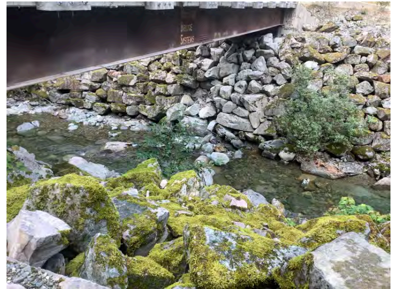
Right Bank Abutment when facing downstream
