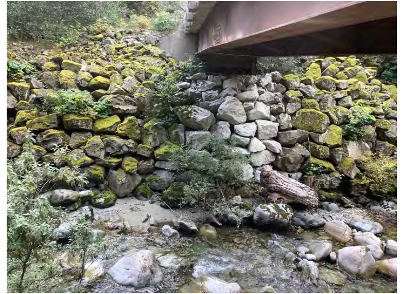
Left Bank Abutment when facing downstream
